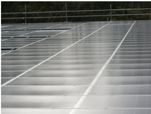
Section of roof showing PV panels
