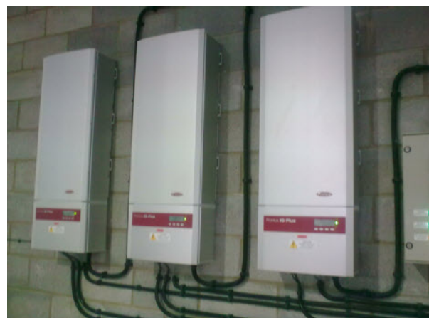
Three Fronius inverters
